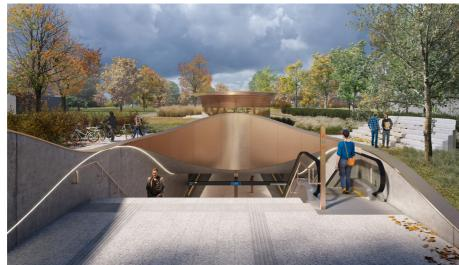
In the design, the daylight voids are designed in such a way that they enhance both the environment and the station, without compromising on their functionality as smoke outlets. Experiencing the full height and seeing the sun or the clouds
